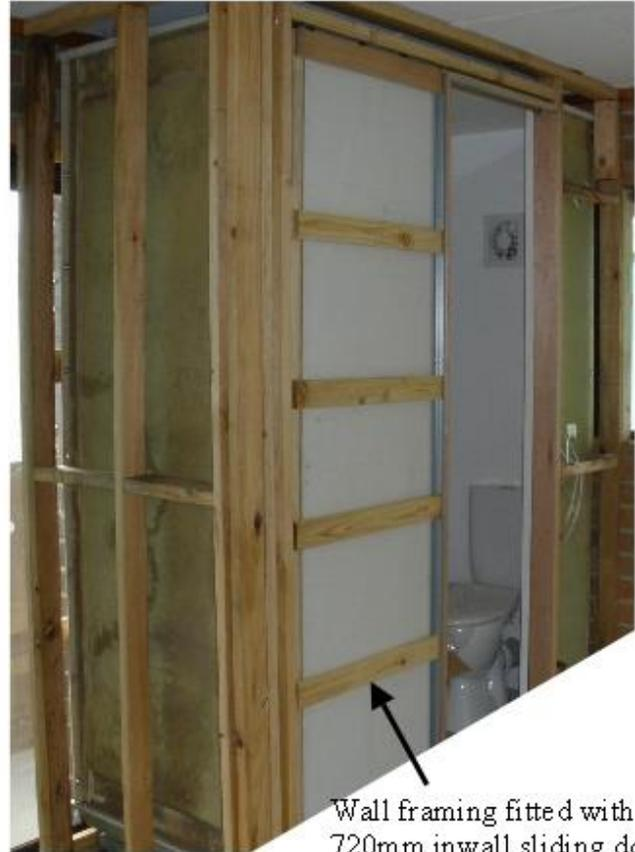
Wall framing fitted with 720mm inwall sliding door.
