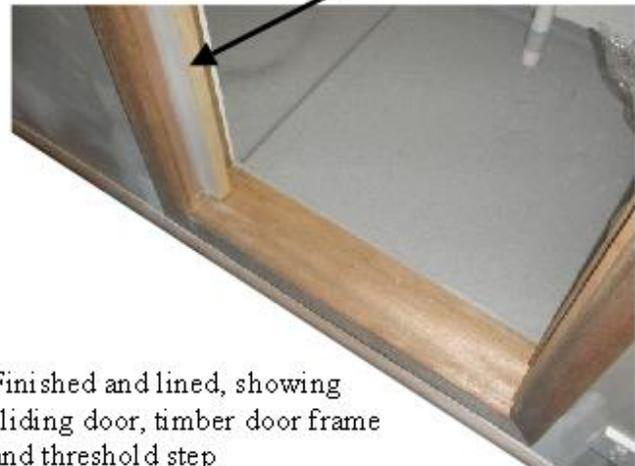
Finished and lined, showing sliding door, timber door frame and threshold step
